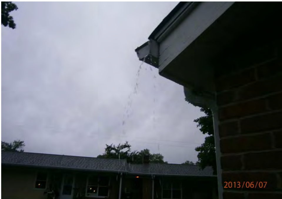
15. Gutter leaking
