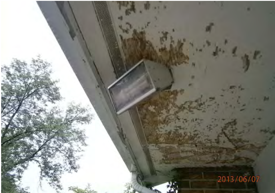
11. Typical soffit peeling paint
